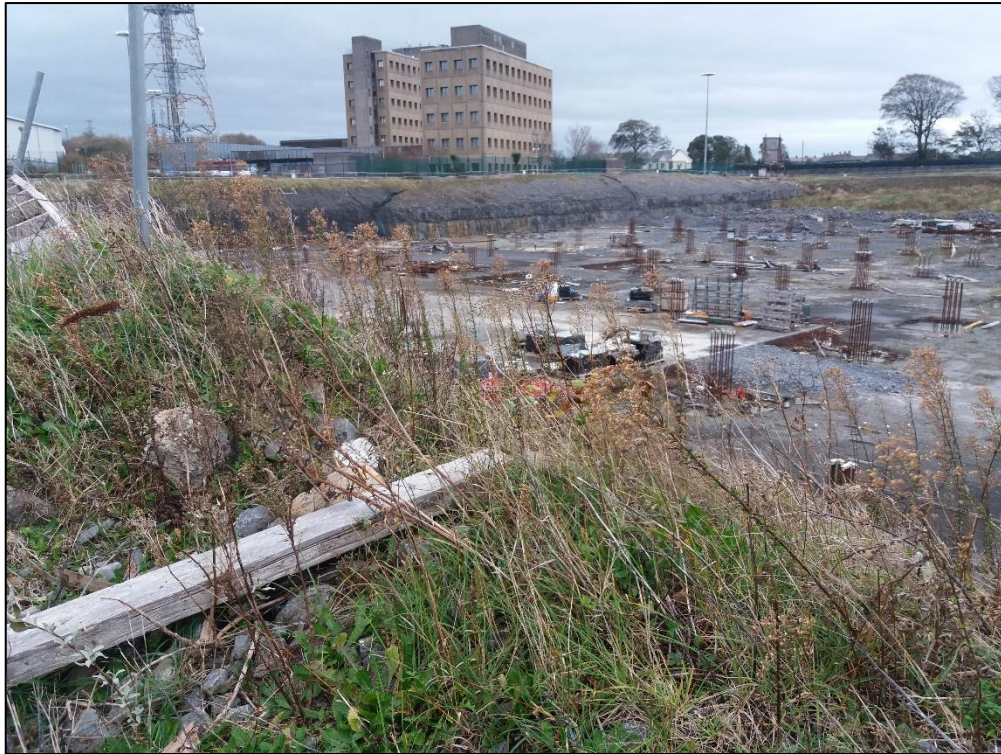
Plate 10.1 View from the north-east of the site looking south-east towards the Eir Building on the Monivea Road. This view shows the extent of the stalled construction works on site. The vegetation present in this image is typical of what is found on undisturbed sites.
