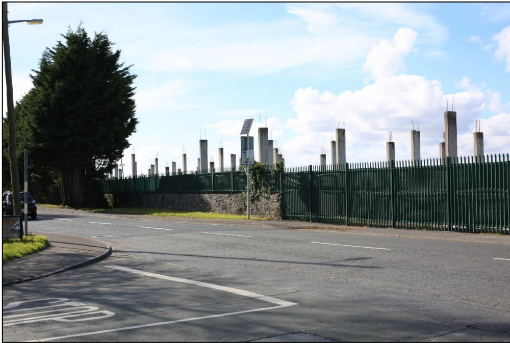
Plate 10.8 – View from the Monivea Road looking northwest towards the site. The site hoarding can be seen clearly from this point along with the existing structure present on the southern part of the site. The large leylandii trees can be seen clearly here, running adjacent to the Monivea Road, screening the western part of the structure.
